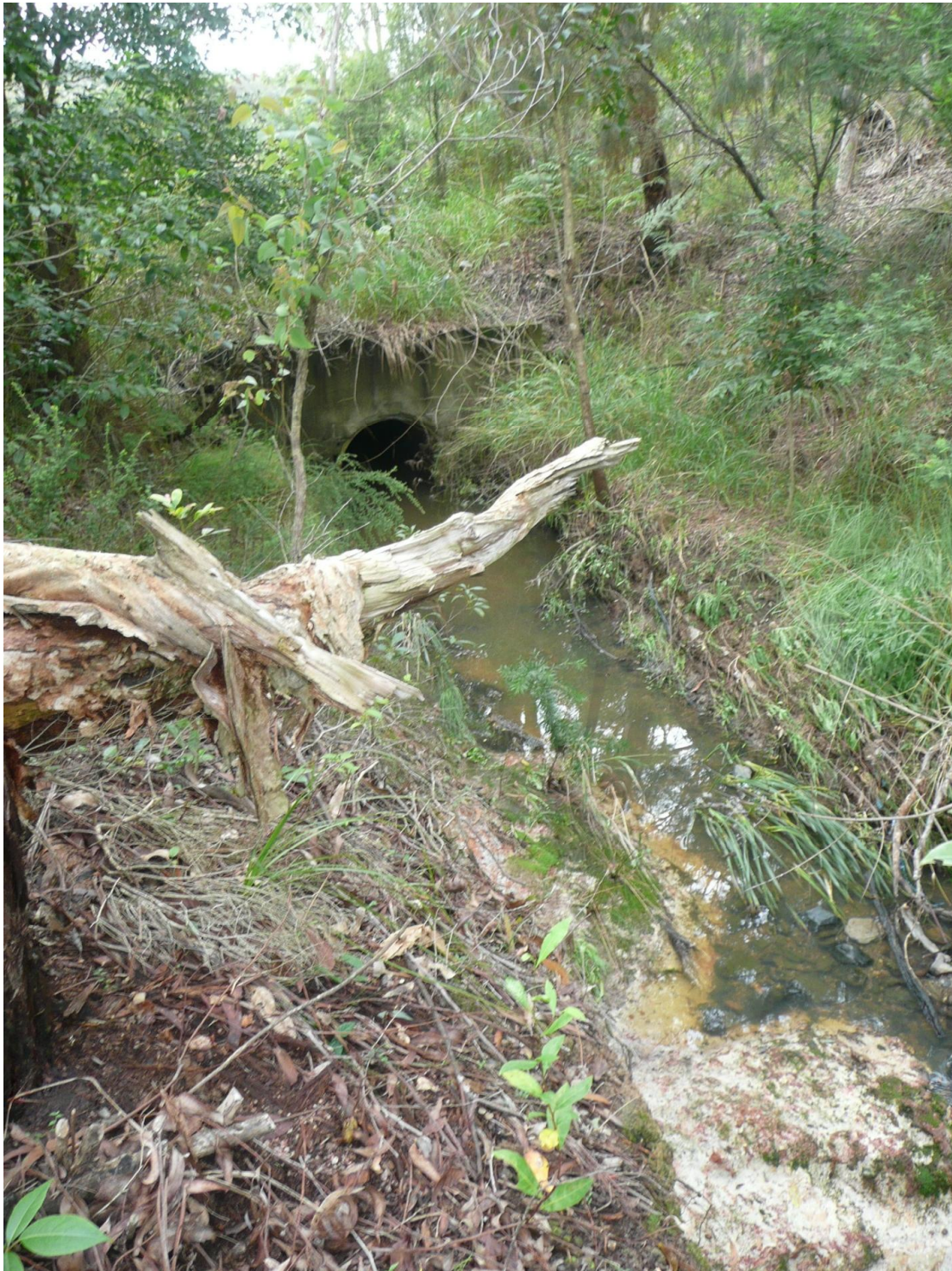
Figure 3.11_Headwall and outlet of Watercourse 2 (Source: HASSELL, 2009)
