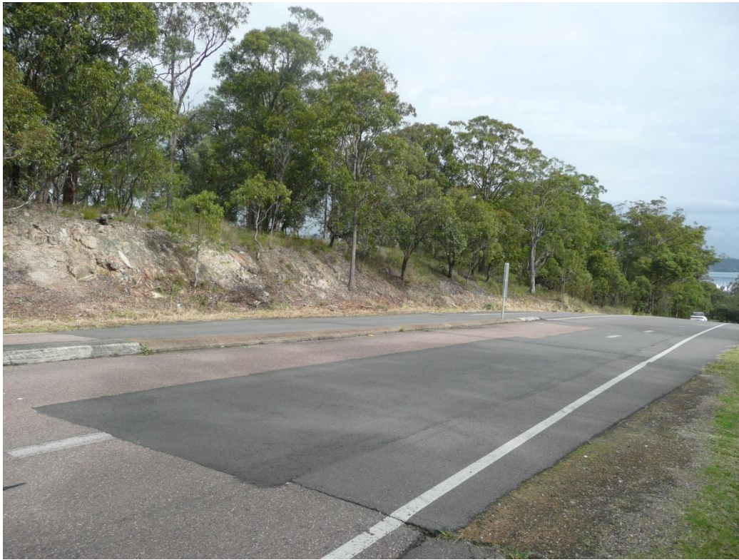
Figure 3.21_Tingira Road, south of the site, looking west (Source: HASSELL, 2009)
